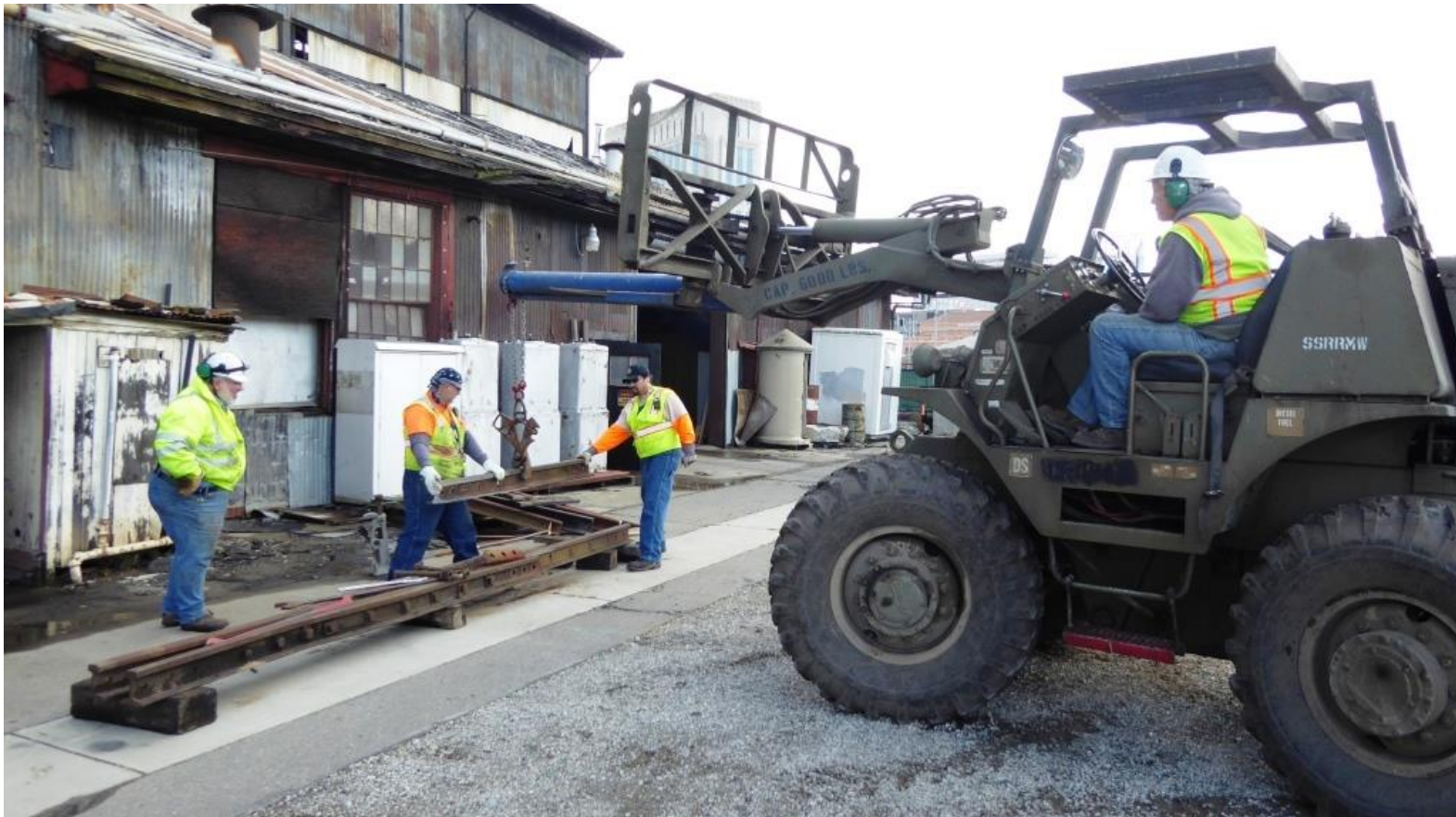
Frank, Mike F., and Jose have Steve on GM2 move the next wing-rail into position
