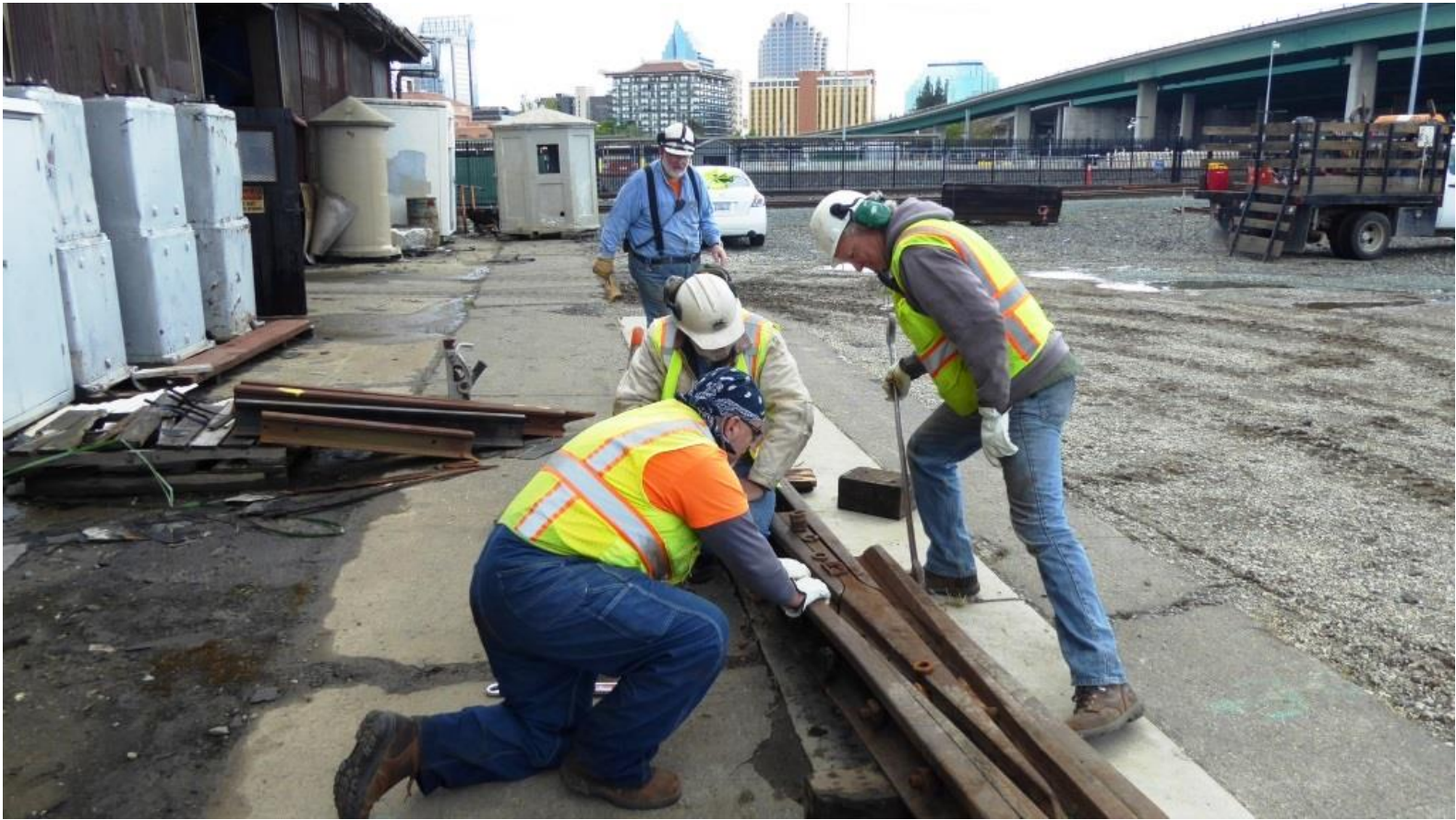
Steve uses a track-wrench to tighten down nuts
