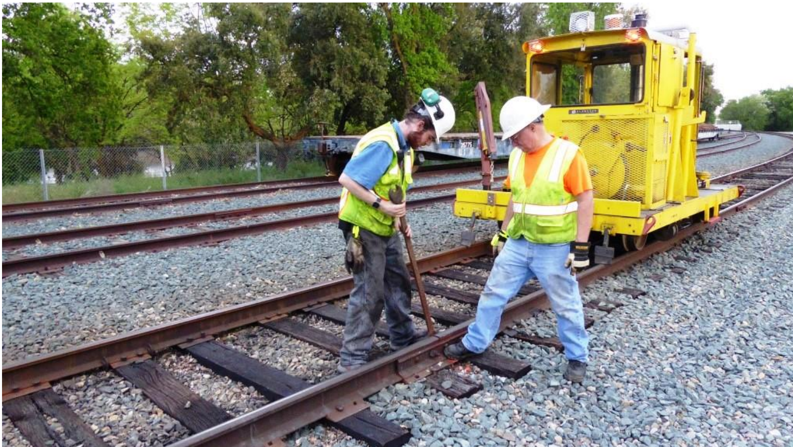
At Baths, Matt and Mike H. replace a broken bolt
