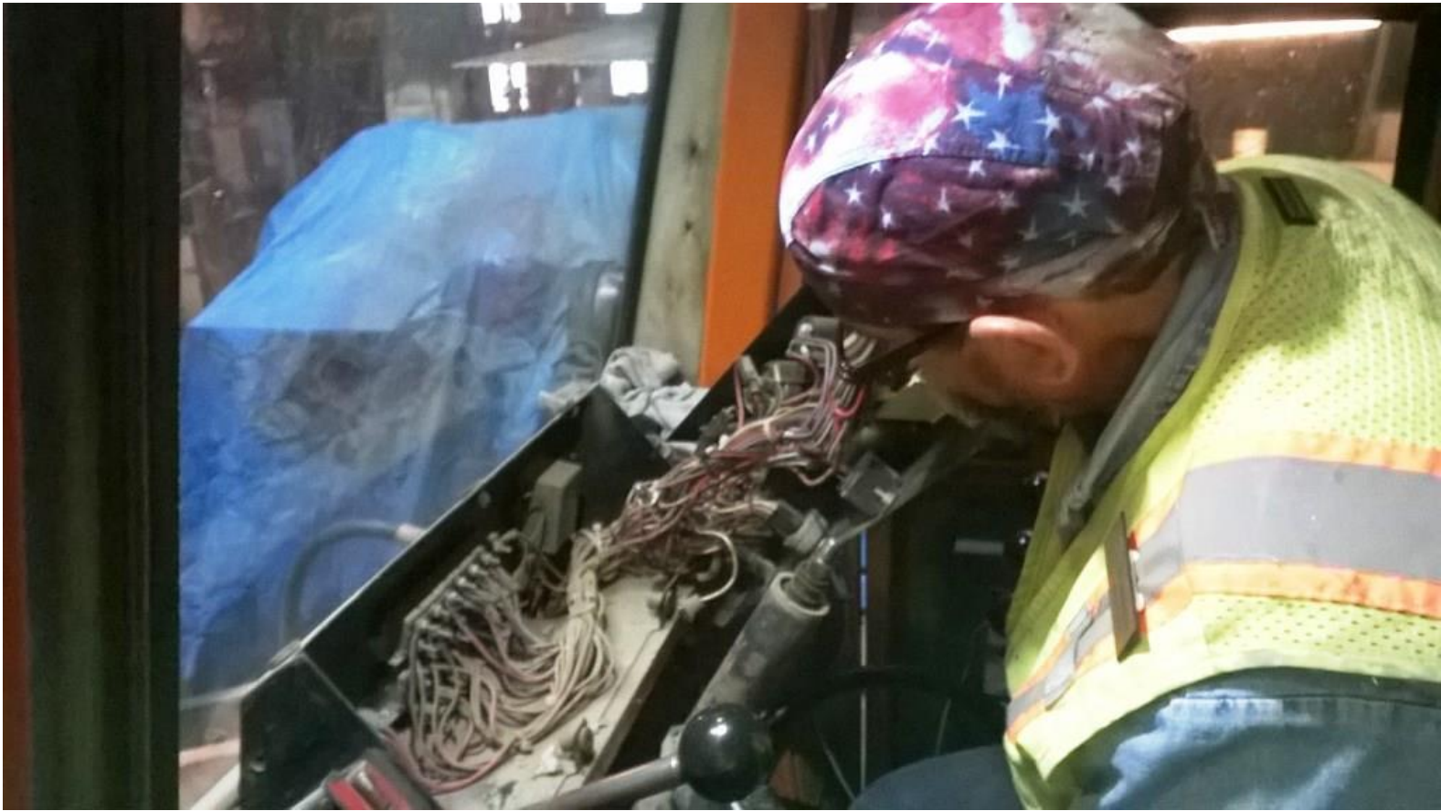
Joe works his way through a maze of wires under the dash of the front-end loader
