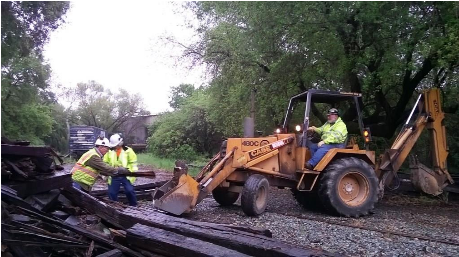
With Frank on the back-hoe, Clem and Ed fill the bucket with dead ties
