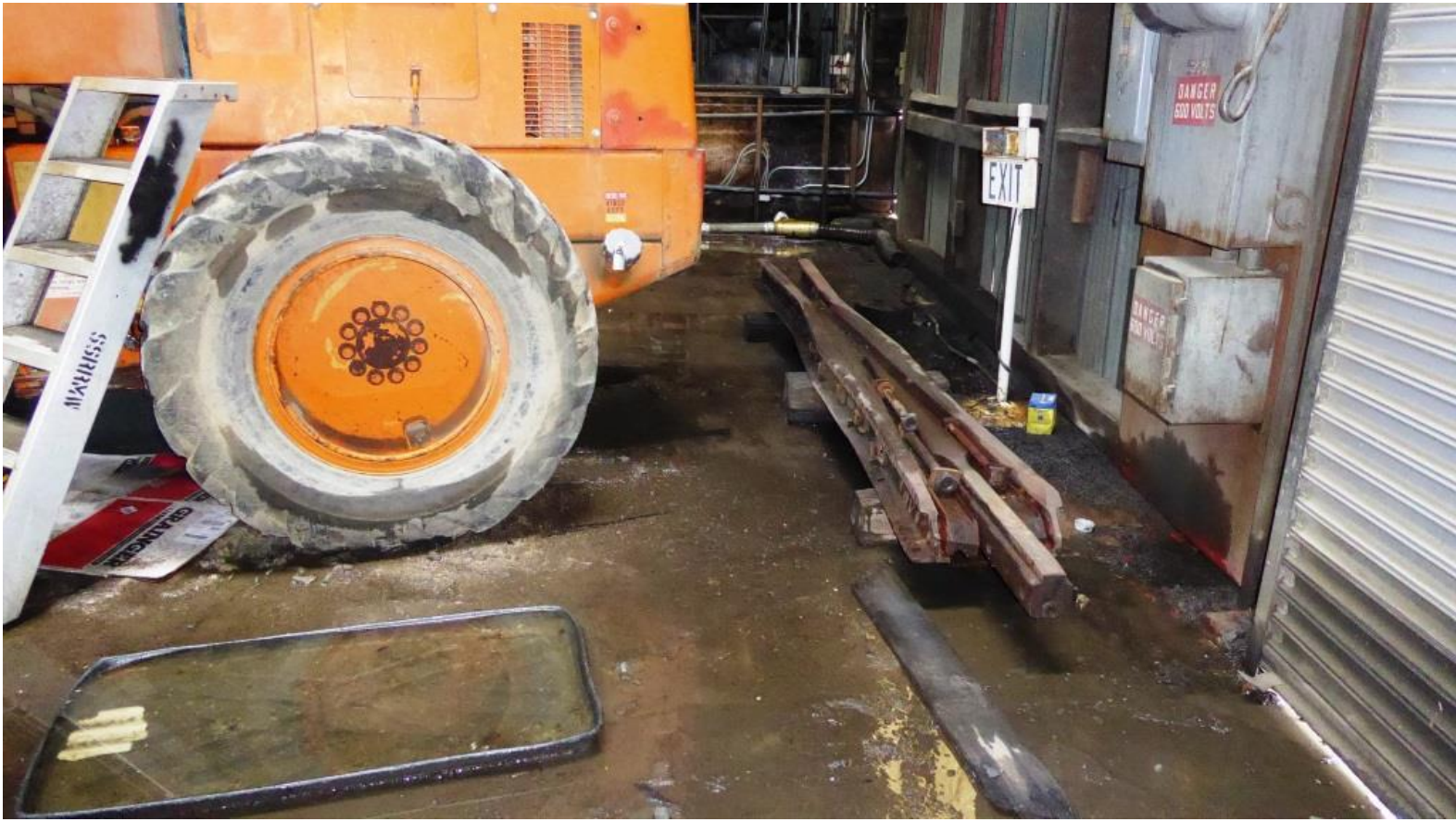
The Switch 19 frog is buried behind the dead loader
