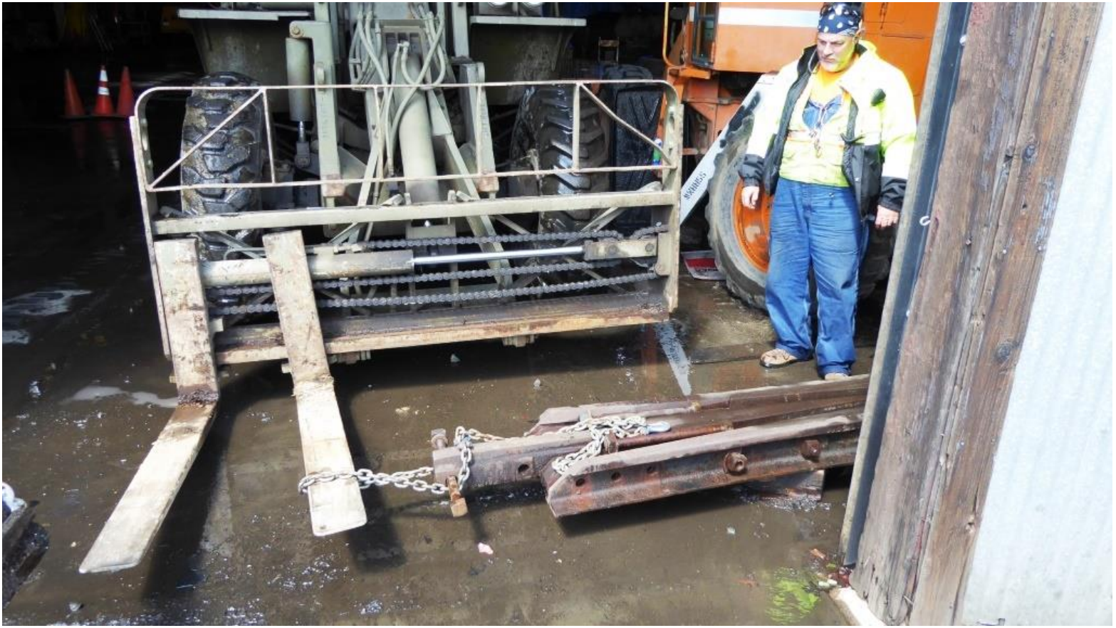
Mike F. chained the frog to GM2's fork which can be moved laterally and pulls the frog out of its hiding place
