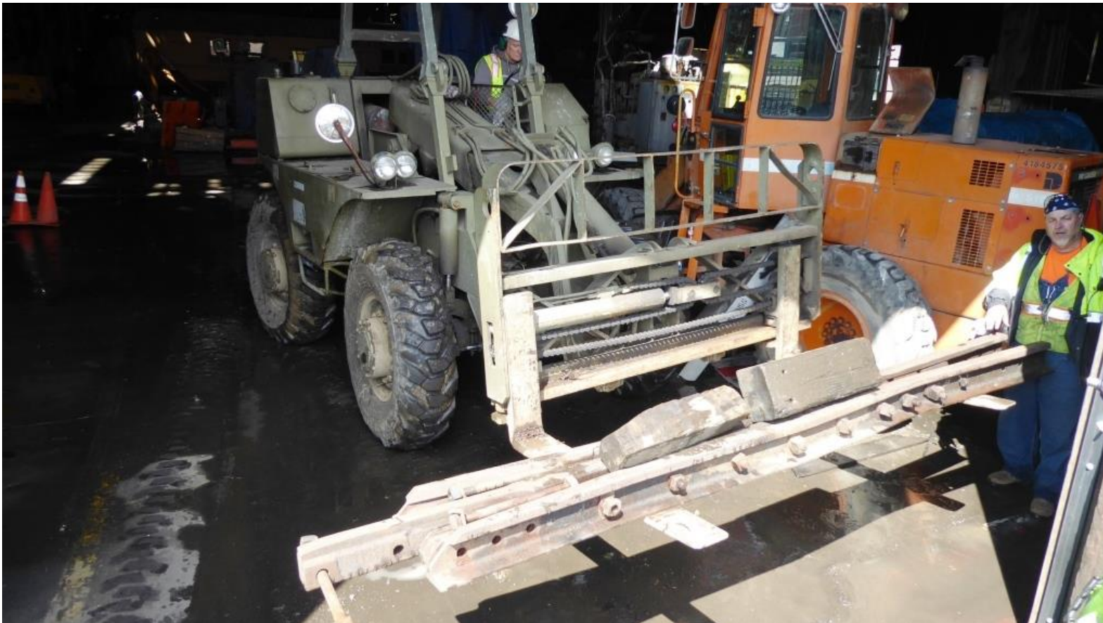
With the frog now accessible, Steve on GM2 lifts it up and prepares to take it outside
