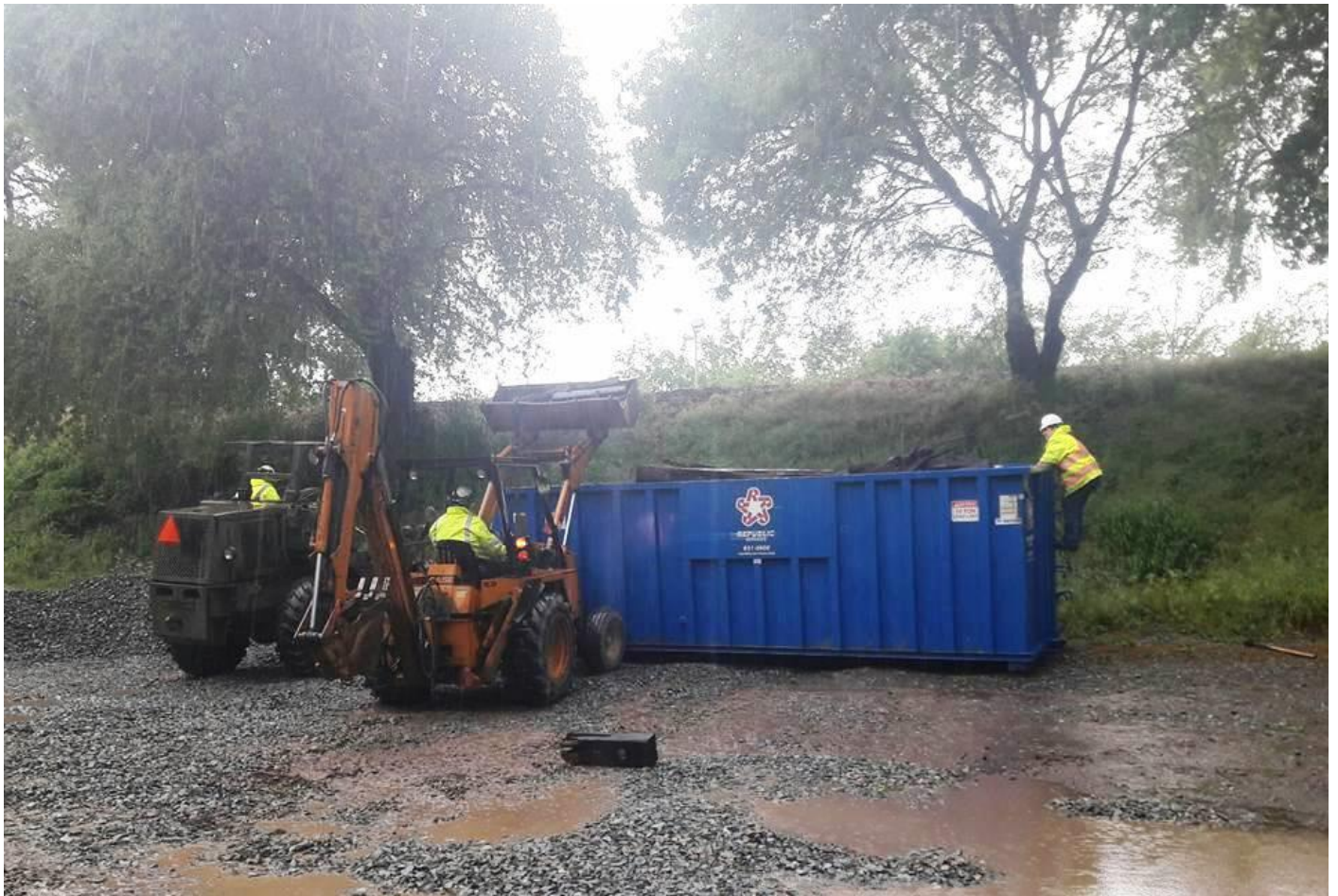
Heather takes a look at how much room is left in the dumpster as Mike F. on GM2 and Frank on the back-hoe dump dead ties
