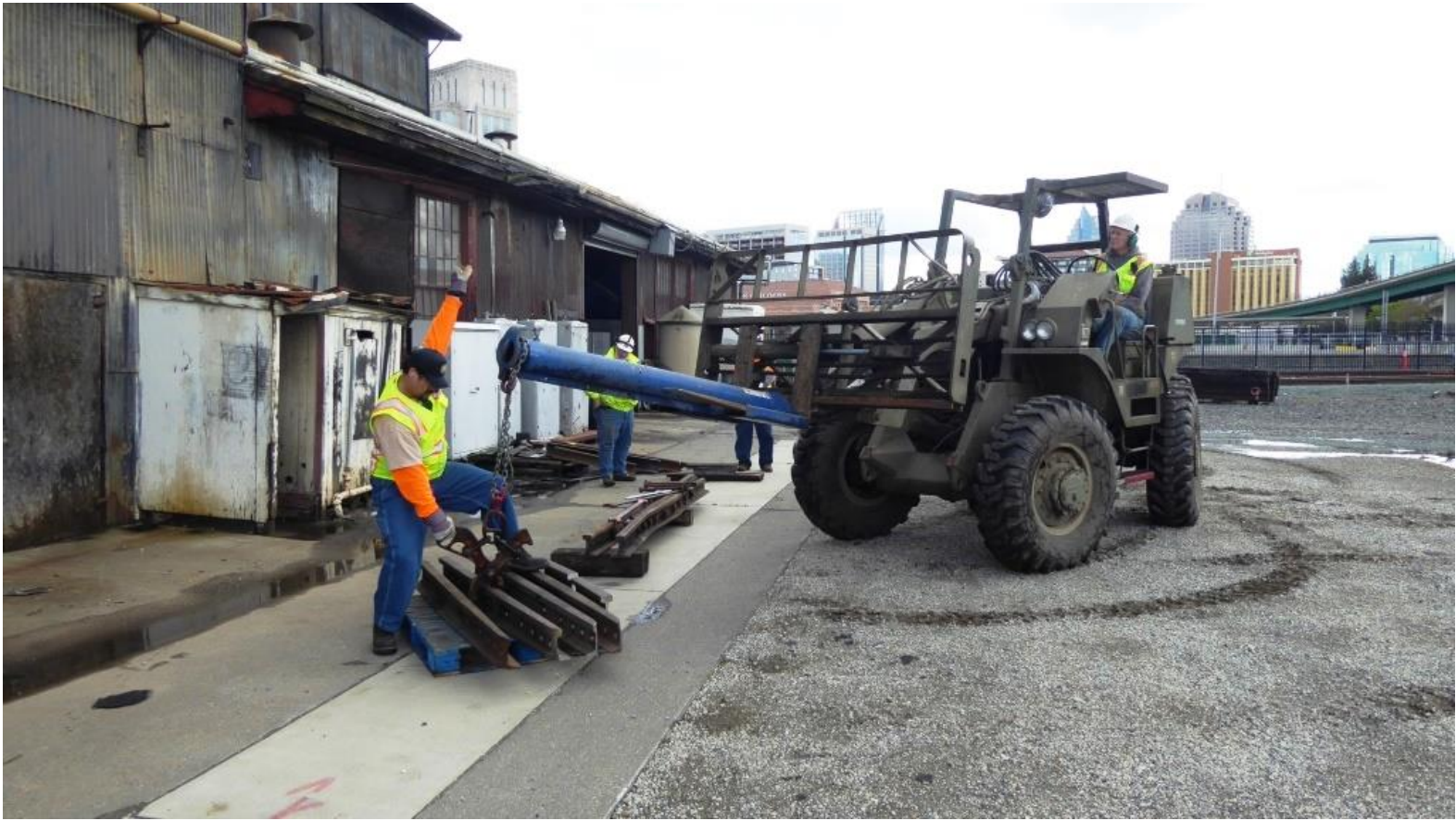
Jose uses rail-tongs to grab a newly milled wing rail which Steve on GM2 will move into position
