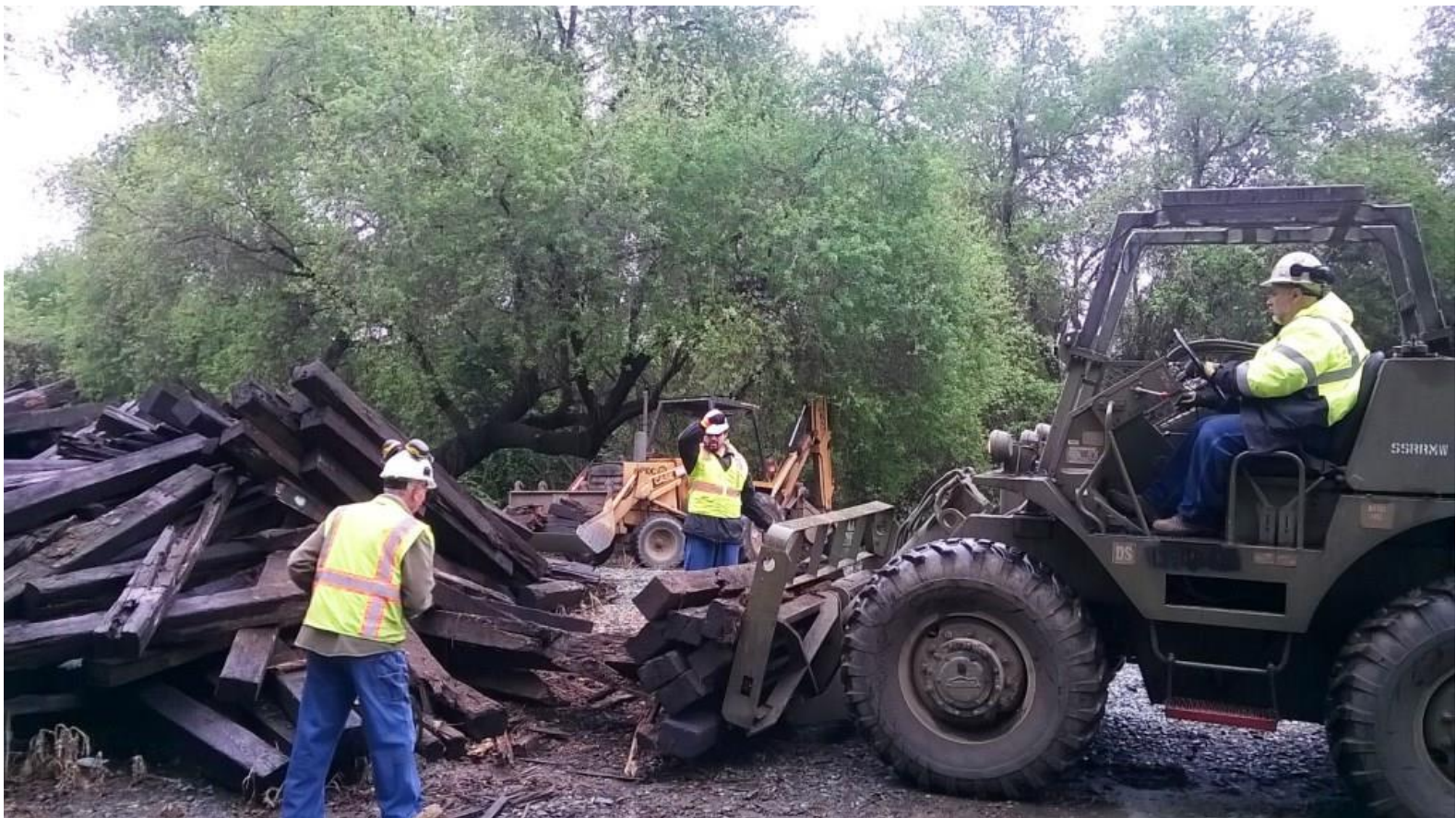
Clem and Jose work with Mike F. on GM2 to load dead-ties onto the forks
