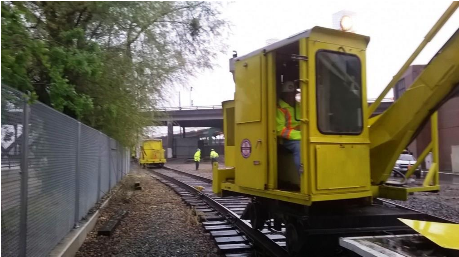
Moving equipment in the rain: Mike H. takes out the tie-crane
