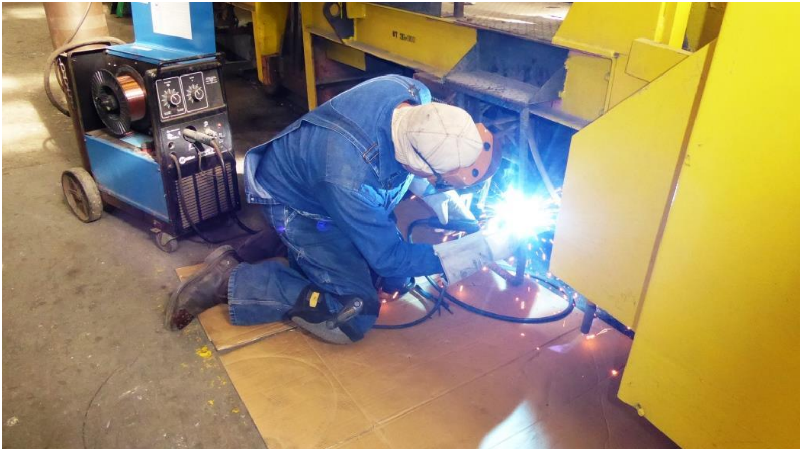
The master of metallurgy, Cliff, welds a new step onto the regulator's rear ladder
