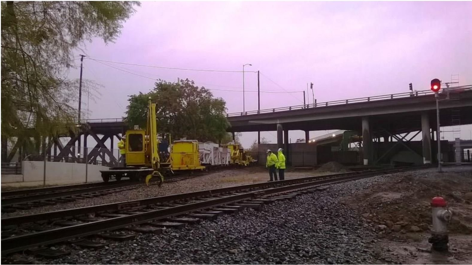
Frank and Ed review their work with the rearranged line-up of MOW equipment
