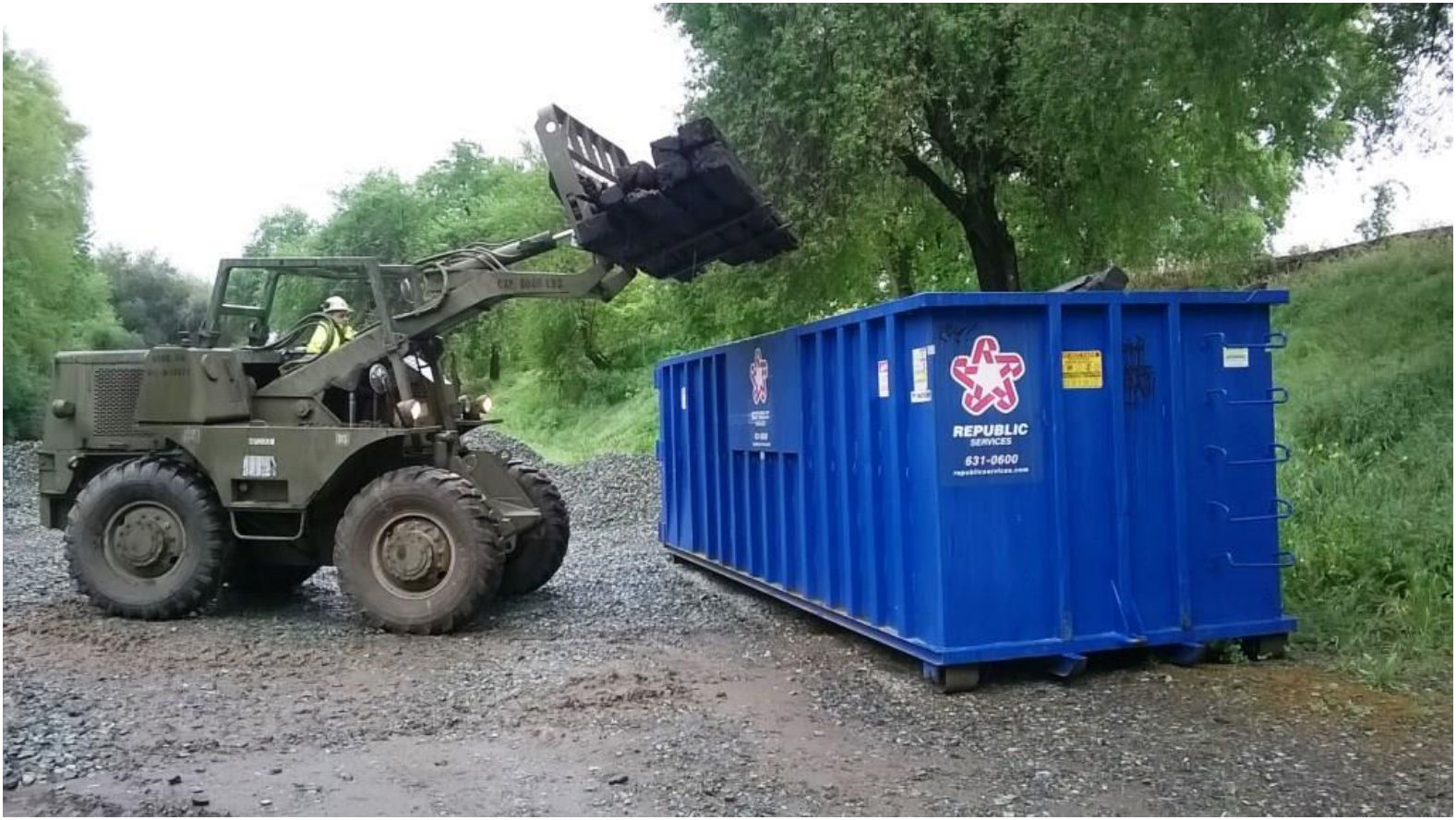
Mike F. drops dead ties into the dumpster
